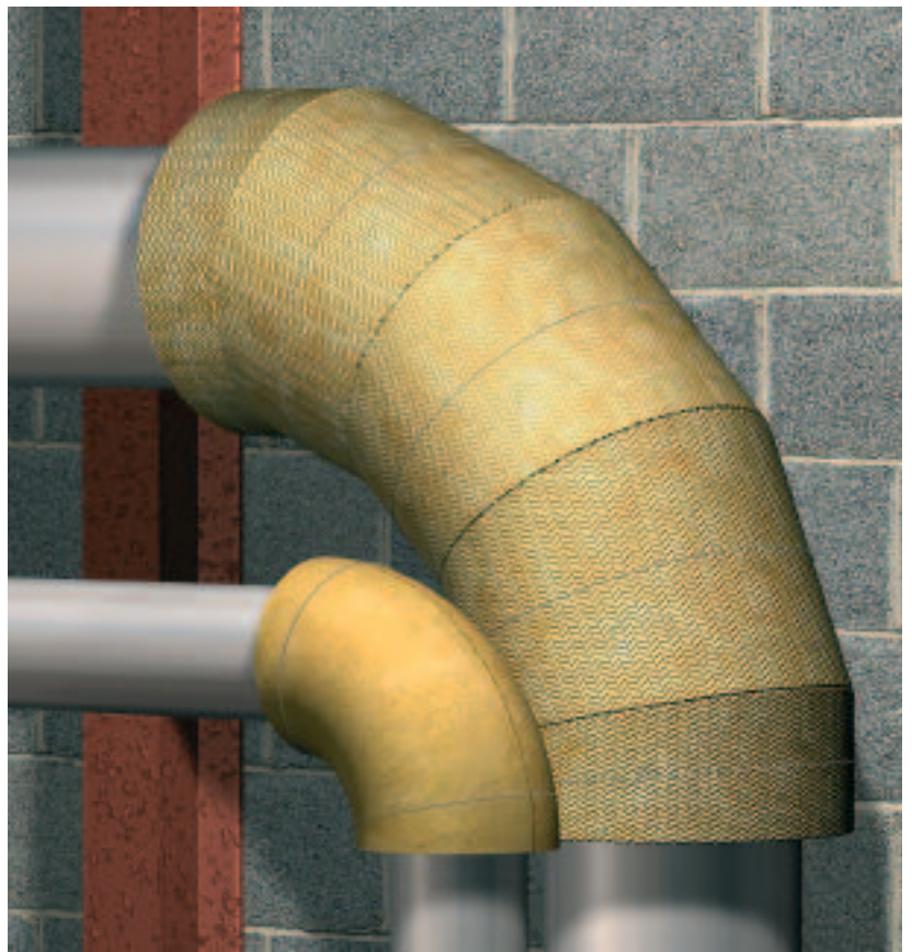
Rockwool Matched-half Bends and Pipe Bend Segments wired onto pipe-work
